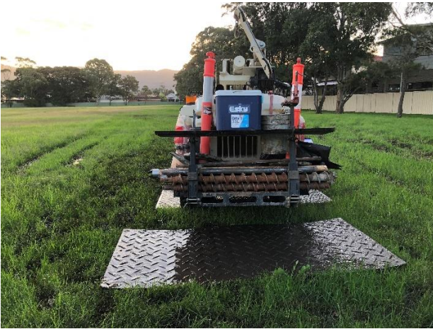
Photo 1 – View of track mats in use, facing west.
